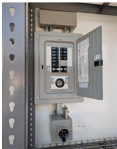
Dual-input load center can accommodate power feeds from the local utility grid or completely off-grid with the use of fuel-based generators, and/or renewable sources like solar.
