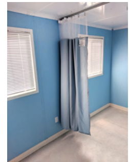
View from interior of exam room, looking toward entrance and waiting area. Antimicrobial, ceiling-mounted patient curtain provides privacy in exam room while creating a waiting area just inside the entrance. Microbicidal paint was used on painted interior surfaces. Continuous welded-seam vinyl flooring is ideal for aseptic applications.
