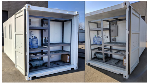
View from exterior at dedicated equipment room that is housed behind the cargo doors of the container. Customer wanted a solution that was highly secure, accessible, and functional. The modular shelving system can be (re)configured to accommodate various mechanical, electrical, plumbing, and communications equipment needs.
