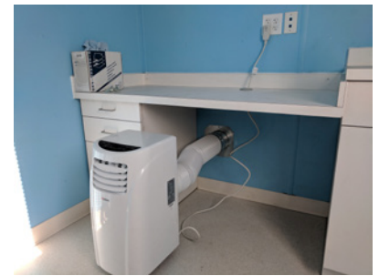
Portable air conditioner unit can easily be connected for use in high-ambient conditions while easily stowed when not in use.
