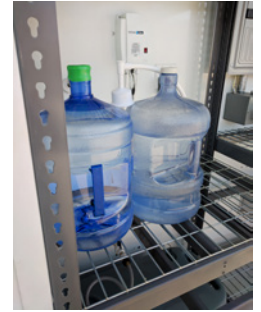
Potable/fresh water supply system utilizes standard 5 gallon water bottles.
